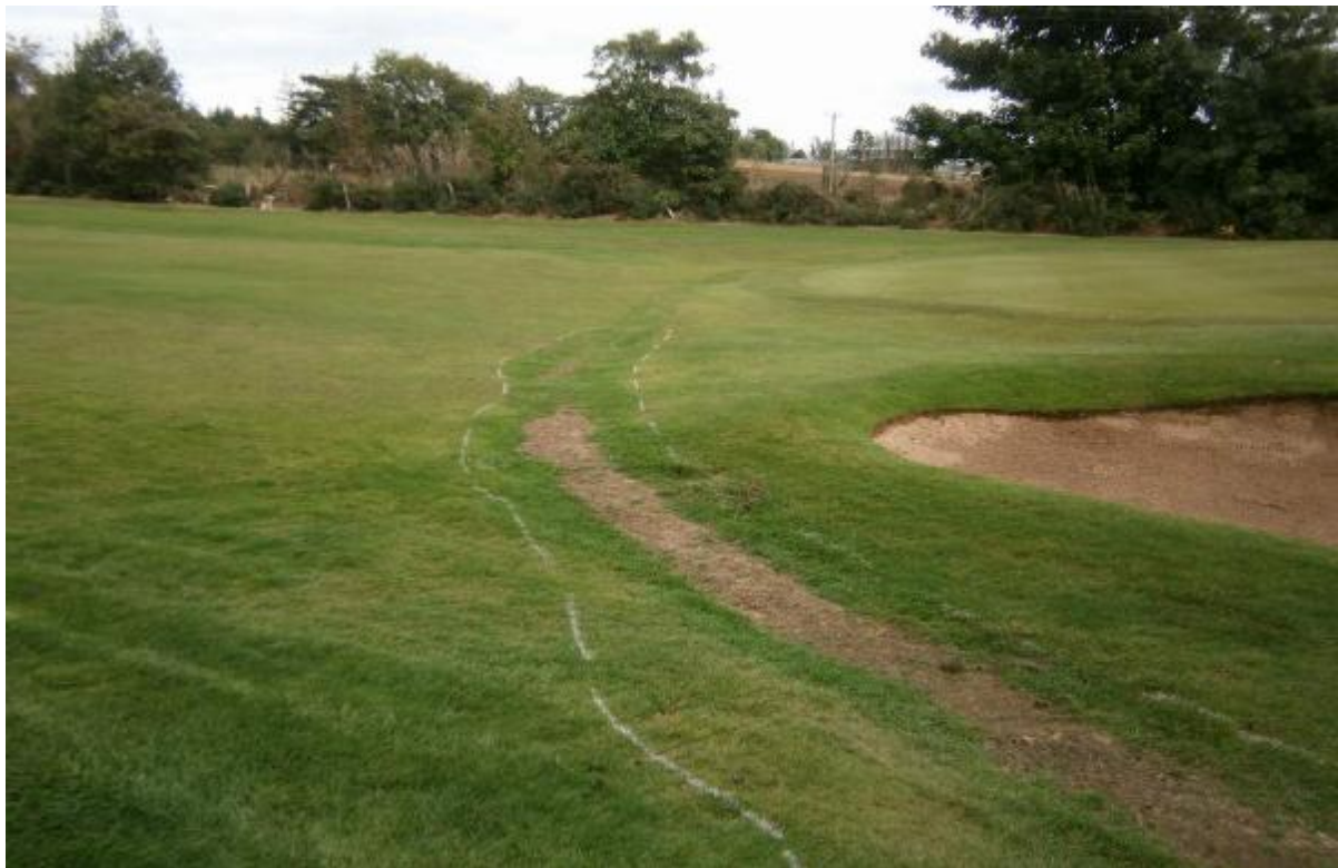
Figure 4 Drainage and gully across the 1 st to intercept surface water flows
